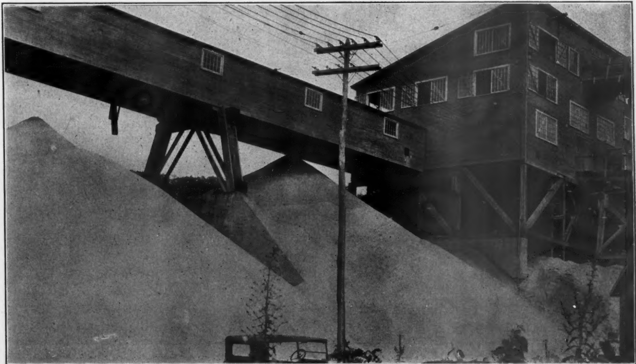
At Top—One of the Primary Crushers, Showing Hand Hoist. Below—Housing for Conveyors Which Drop Material on Storage Piles
